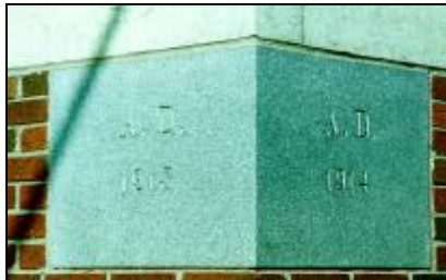
A cornerstone joints two walls of a building together and is generally the first stone laid in the wall of a new building. A cornerstone points to the visible support upon which the rest of the building relies for strength and support.
